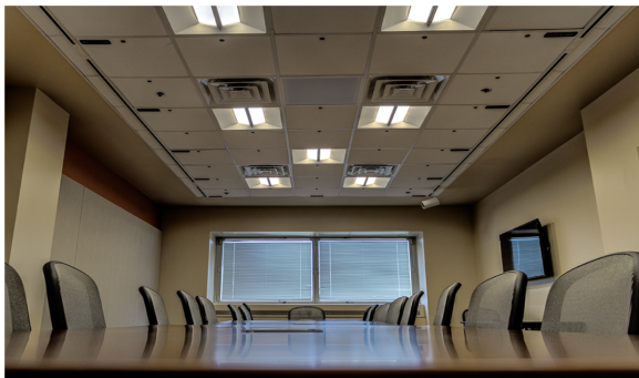
Figure 2: The Smart Conference Room at Rensselaer. The black dots in the ceiling tiles are RGB color sensors, and the black bars are infrared time-of-flight sensors.
